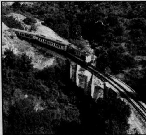
The current state of Israel's rail system is in vital need of modernization. Israel Bonds investment dollars are helping to build a new system of high-speed railways connecting Tel Aviv to Beersheba, linking the heart of Israel's urban centers. Photo by John Wagner.
