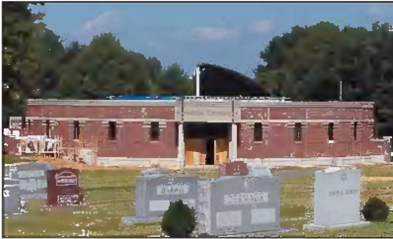
The nearly-completed cemetery memorial building.
