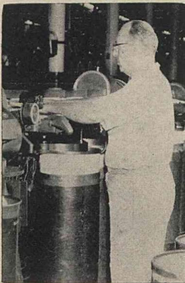
DAVID LOWERY, drawing tender, makes an adjustment on a drawing frame. At this stage several sliver ends from the preceding carding process are combined and drafted out so that the resultant sliver is the same size, but more uniform, than the original.
