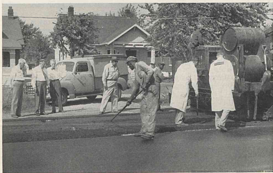
CONTINUING ITS LEADERSHIP IN THE DEVELOPMENT OF RUBBER ASPHALT ROAD AND PLAYGROUND SURFACING MATERIALS, THE COMPANY ANNOUNCED A NEW LOW-COST, SYNTHETIC LATEX COMPOUND DIFFERENT FROM ANY RUBBER HERETOFORE USED IN ASPHALT ROADS.
