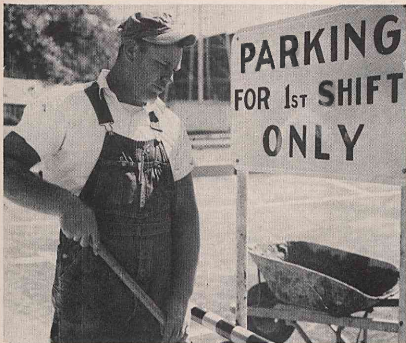
FOREST DELLINGER, Shop, places one of the permanent signs in the new Company parking area between Franklin and Second Avenue. The parking lot, now in use, is of much benefit to the increasing number of automobile owners employed by the Company.
