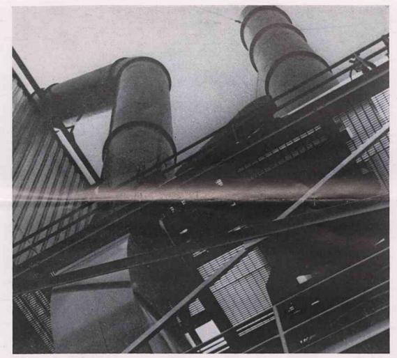
• Portion of the Gastonia Firestone Textiles Company equipment installed in 1972, to capture and clean smoke and fumes at one of the largest cord-treating units in the textile-rubber industry. The huge electrostatic precipitator is the first of its kind to be operated in the tire fabrics field. A similar unit will be installed at the di-
