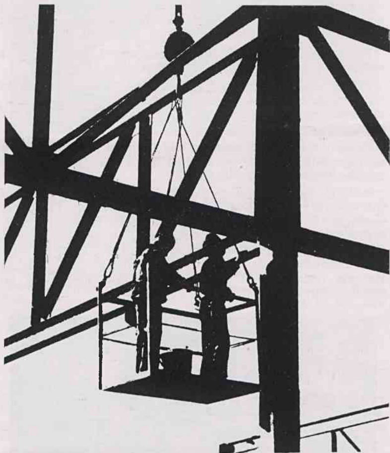
Two workmen connecting beams high above the Knoxville 1982 World's Fair site.
