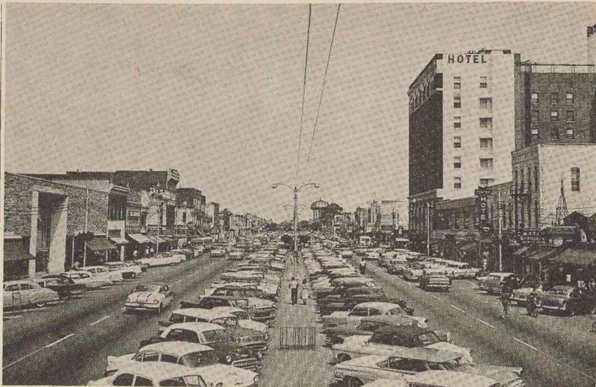
Goldsboro's main thoroughfare can be seen above. The strip in the center of the street used to be the bed for railroad tracks, but in 1924 a group of determined merchants was responsible for their removal (see story). The city has been termed the shopping center for Eastern North Carolina, or as one wit put it, "the golden buckle on the tobacco belt."
