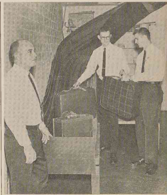
Agents Ronnie Abshire, Darris Moore, and Jim Birthisel collect bags sent via the baggage chute from the ticket counter upstairs.
