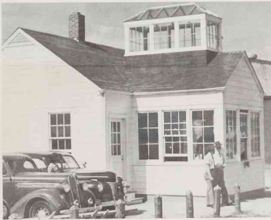
This was the operations building for the Civil Pilot Training (CPT) and War Training School (WTS) programs. Employees built the cupola on top for use as a control tower.
