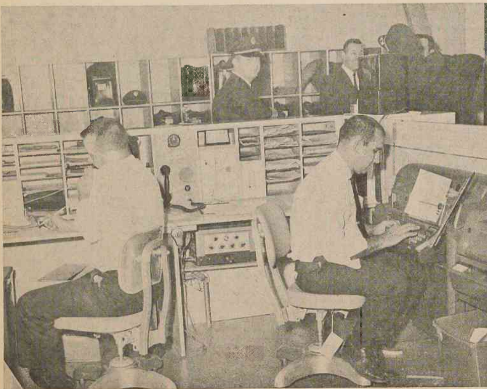
NEW OPERATIONS HEADQUARTERS — Agents at Washington National have moved into their new facilities. Already hard at work are Ron Rush, at left, and Tom Cleghon. Flight crews ready for departure are in the background.
