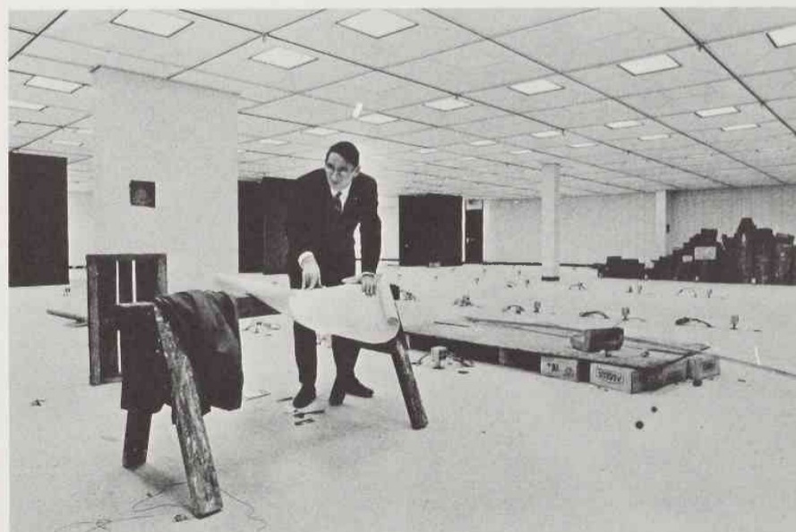
THE MAN MOST FAMILIAR with the new CRO, at least at this point, is Vice President Bill Barber who has been in charge of the building's actual construction. He is standing in the main area of the building, where the agents stations will be located.
