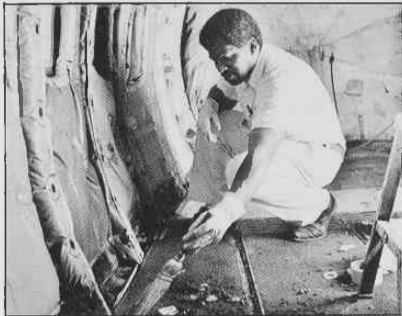
John Wiley, Maintenance cleaner, brushes out dust as well as other debris from the wainscot panels.
