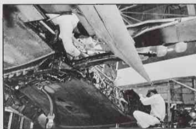
Sheet metal repairs in the flapwell area of the wing are made by mechanics Steve Guidry (foreground) and Vernon (Buzz) Basham.
