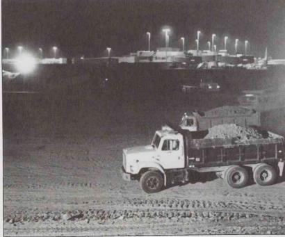
A half million cubic yards of dirt have been brought in at CLT to build up the area at the end of our concourse. The city will soon begin paving and preparing the ramp and taxiway for service. The work
