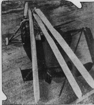
a ride around the countryside. Uncle Sam is furnishing the financial backing for the development of a low cost wingless plane of the gyro type, with rotor wings that fold back. Here we are looking down on the folded rotors. The plane embodies most improvements of the safety type and eliminates many things that have kept the average man from
