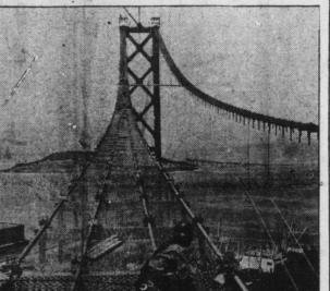
Here are seen men working on the catwalk of the San Francisco Oakland bay bridge extending from the San Francisco anchorage to the central anchorage near Yerba Buena Island. The catwalk is made of four two and one-quarter inches in diameter with what looks like magnified chicken wire slung between them. The cables from which the bridge will be suspended will be spun three feet above the catwalk.
