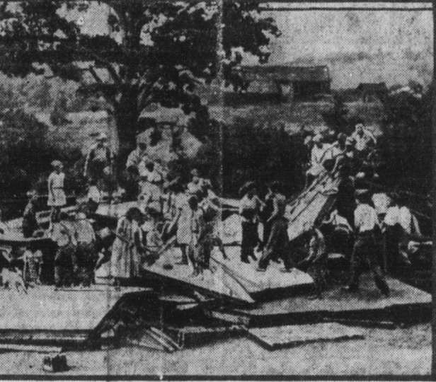
Any wind that blows down a school house is all right, according to the children shown in this picture playing in the ruins of a portable school at Bairdford, near Pittsburgh, Pa. A sudden gale blew the building a hundred feet from its site and effectually flattened it.
