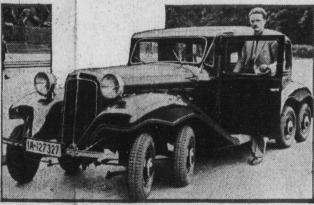
Herr Gotthardt Rimmek, Berlin automobile engineer, is shown here with the new eight-wheeled passenger car which he has designed. He claims that the car offers greater security and is better equipped to take bumps. He explains this by the fact that the wheels of the car do not go through the depressions, but pass over them. Furthermore, a breaking of the axles or a blow-out of a tire will have no serious effect since the car will continue on seven wheels.
