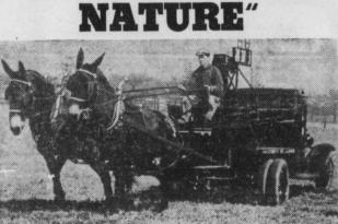
Mighty Mules Hitched to a dynamometer (a strength testing bine) these powerful mules record their strength for the photographer.
