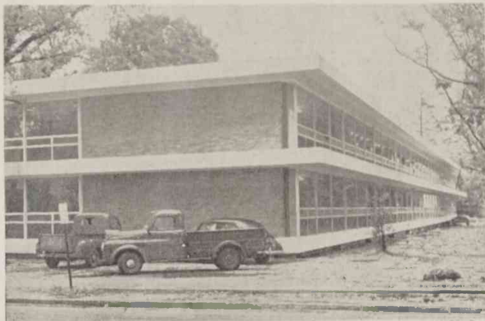
Pictured above is the new classroom building designed to accommodate a student body of 1500 students. There is actual seating space for 850 students at any one time in the building and room for faculty offices for all departments except science, math, music, and physical education.
