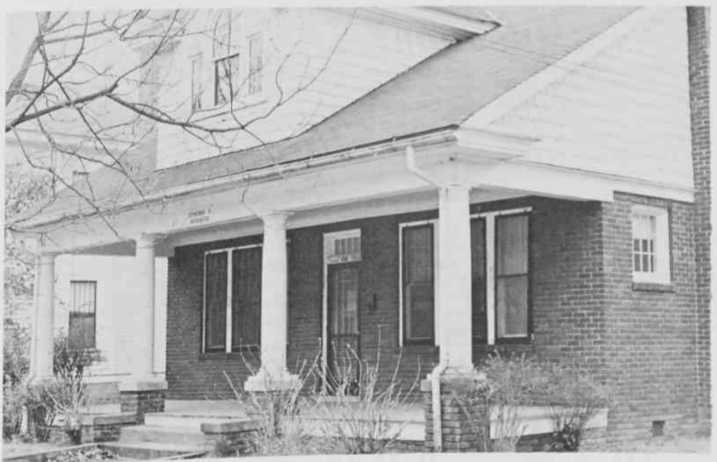
A few of the houses that front Lee Street are beginning to be destroyed to make way for the new library. The two frame houses up the street from the faculty parking lot have already lost their lives. Demolition began in earnest this past Tuesday as workmen merely rammed a bulldozer into the side of the first house, knocking the foundation apart.
