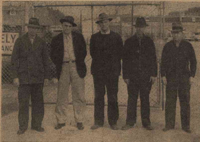
These men are constantly on the job all over the plant and grounds, watching for any emergency condition. Reading from left to right, they are: Cad Whitmire, Alvoid Galloway, Harris Jones, Jessie Allison, Clarence Greene. Two watchmen were not present when this photo was made and they are Yancie McCrary and Alfred Beddingfield.
