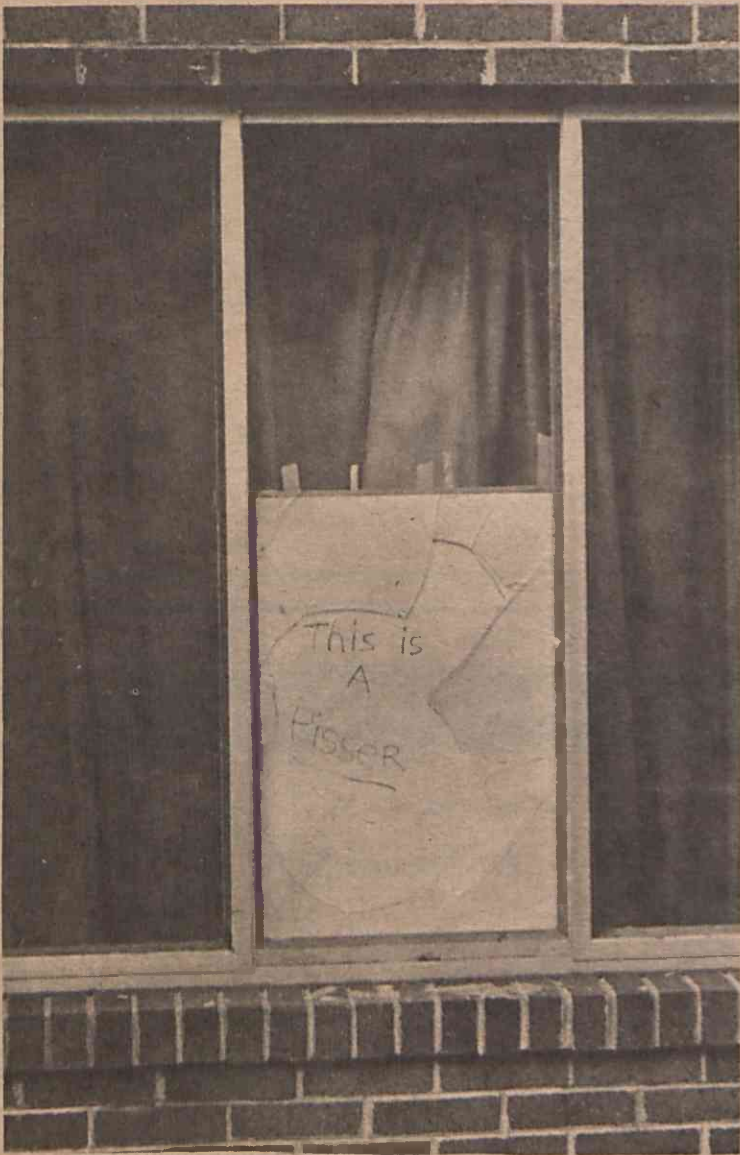
An appropriate message for almost everyone concerned is scrawled on this makeshift repair for one of the damages that caused the ouster of Curtis White as Dormitory Proctor of I Dorm in recent Administrative reprisals.
