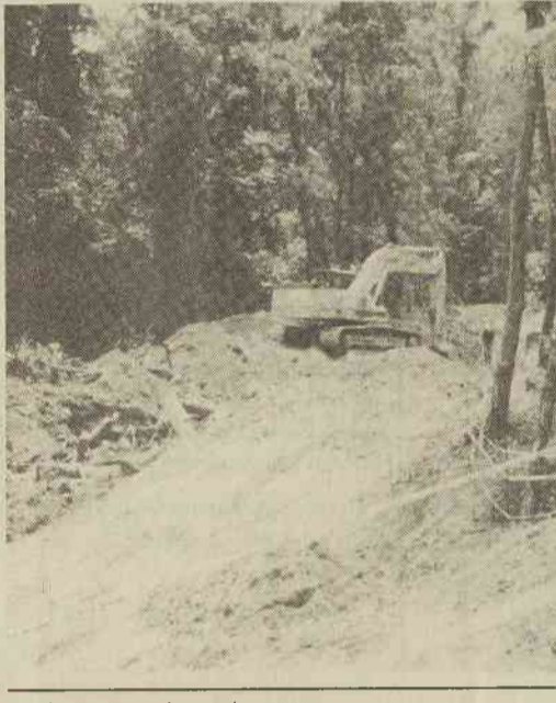
Road construction began this summer.
