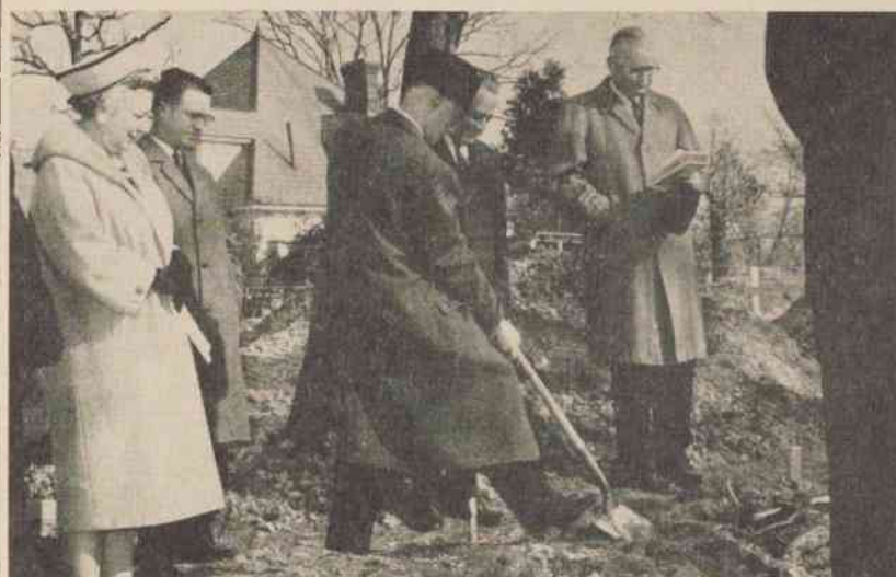
Groundbreaking for new dormitory
