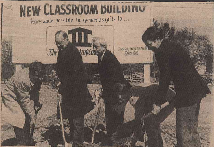
Norris, Taft, Jorden, Smith, Ricketts break ground.
