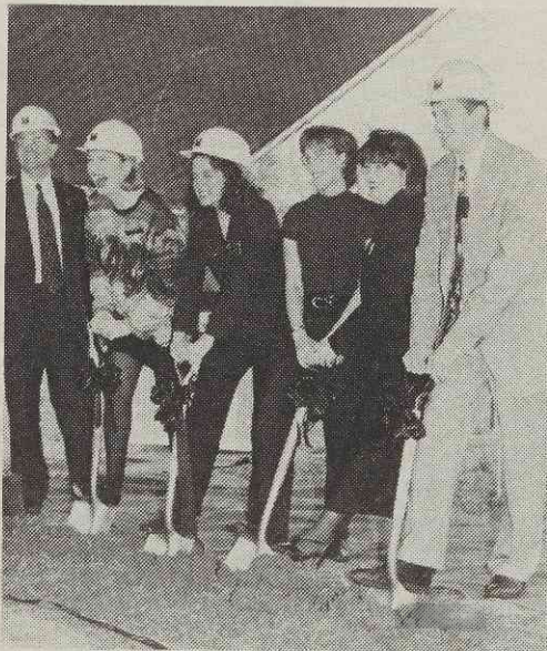
Gardner-Webb President Chris White and various dignitaries break ground on March 19 at the future site of the University Commons Apartments. The apartments will be completed by August.
