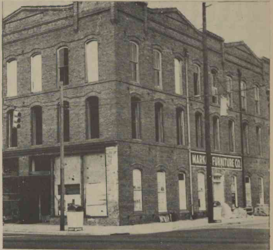
The Old Market Furniture Building yielded a great many artifacts from Scotland County at the turn of the century. St. Andrews Professor Margaret Houston supervised the four-week excavation.
