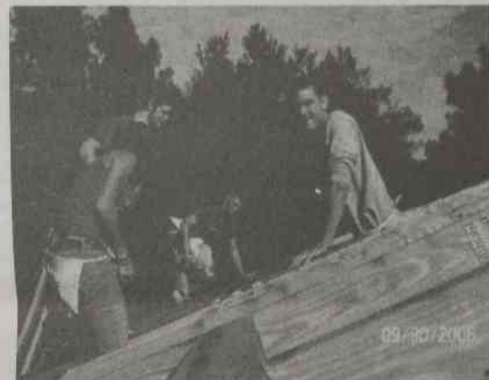
Students working on Habitat House. Courtesy of Reid Mosher
