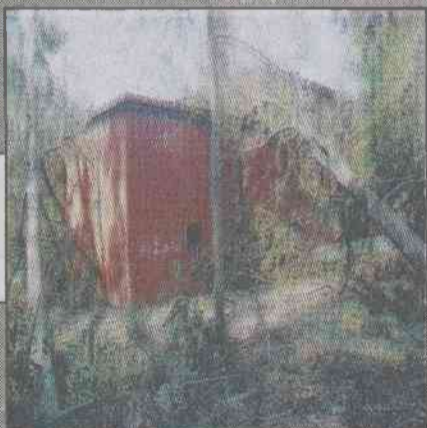
Fallen trees were the major source of damage to buildings.
