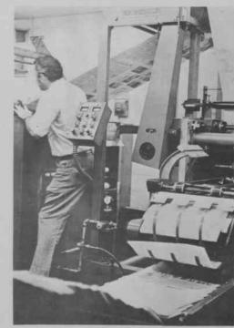
Finally, the job is printed. Two or three pressmen must keep constant vigil over ink, paper, etc. The press prints on both sides of the paper, then cuts and folds it.
