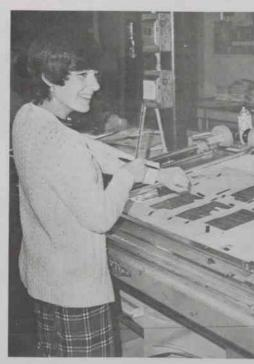
Then the "stripper" tapes this negative to a sheet of paper called a flat. Then he cuts a "window" in the flat, so that all of the letters are showing.
