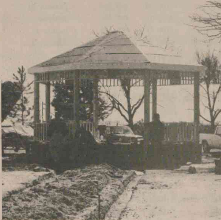
Gazebo-Chowan Campus new edition. Still under construction.
