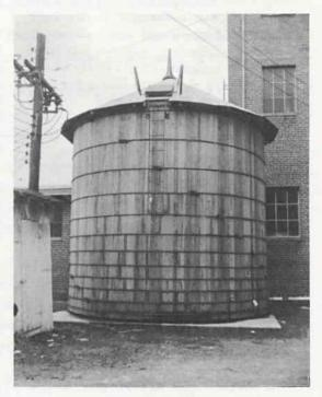
The new 20,000 gallon capacity tank at Plant #4 supplies water for the dye house. Water is pumped from the plant's own deep well and the city supply in Kernersville. The use of this tank enables the plant to use their own well and to store water from the city supply, thereby furnishing an ample supply for the dye house without creating a shortage in the remainder of the plant.
