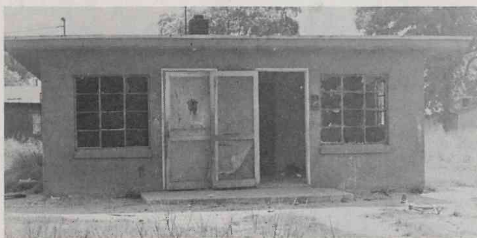
Above, Farmington Forest Apartments, where the Allen Hayes family now lives; below, the remains of the Charles Bennett home at 501 Loflin Street, which is marked for demolition. The family of eight previously occupied the three rooms on the right-hand half of the duplex.
