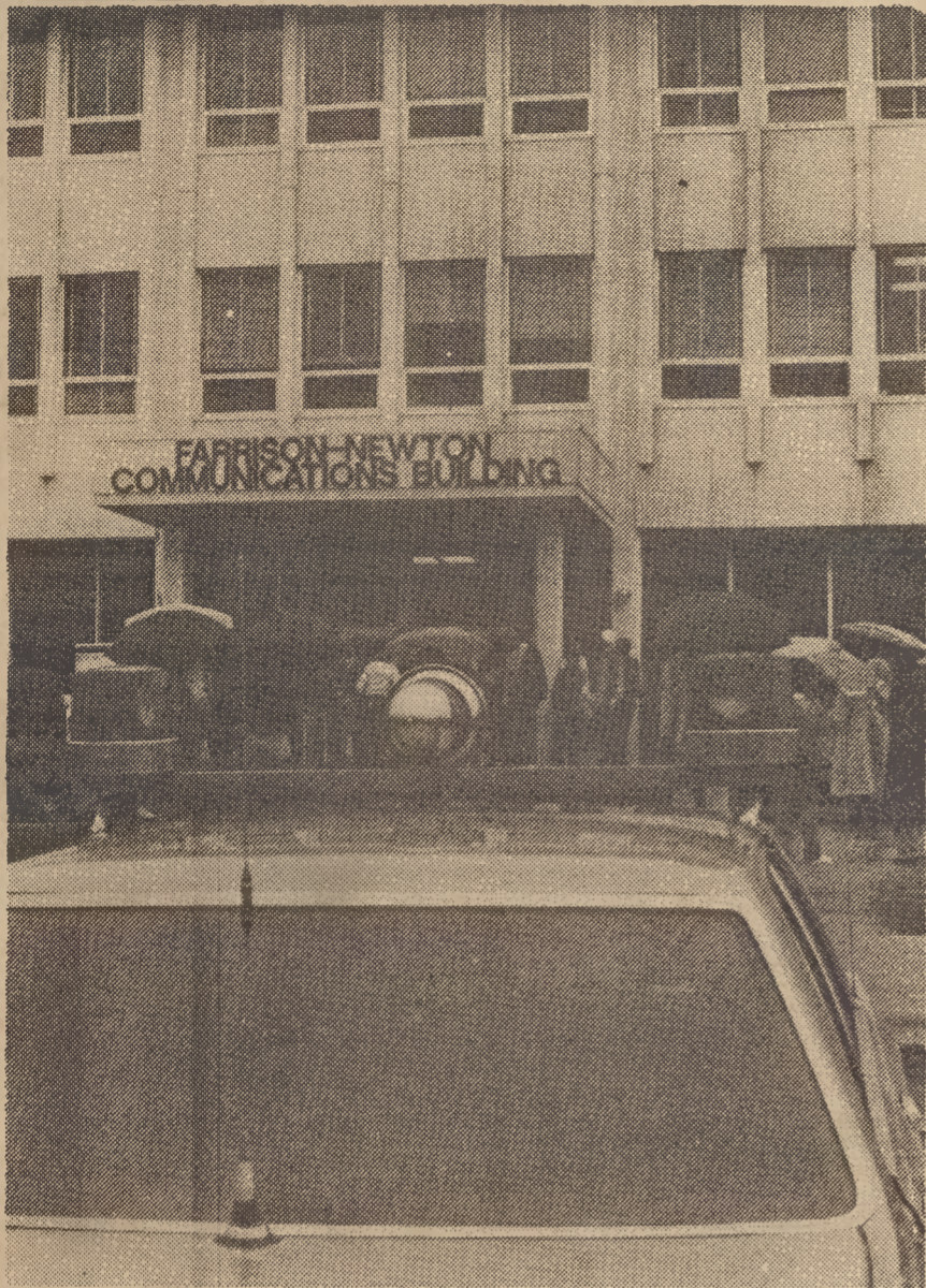
Evacuating a building correctly means never having to say you're sorry.
