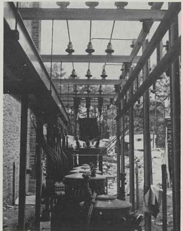
Right: Electricity is supplied to the new building through this transformer station.
