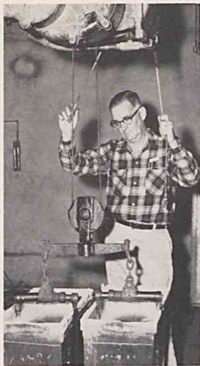
Mr. Rufus B. Carr, Hospital Ice Plant operator since 1952, uses a pulley to draw up two frozen blocks of ice (300 pounds each) from their "briney bed." The brine circulates around the ice blocks (which are contained in cans) and keeps the blocks frozen until they are "pulled."
