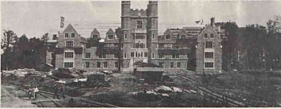
DAVISON BUILDING IN 1929 — The medical school building, later named for Dr. W. C. Davison, the school's first dean, was the first facility constructed in the now-expansive Medical Center complex. In the foreground are railroad tracks used to deliver construction materials.
