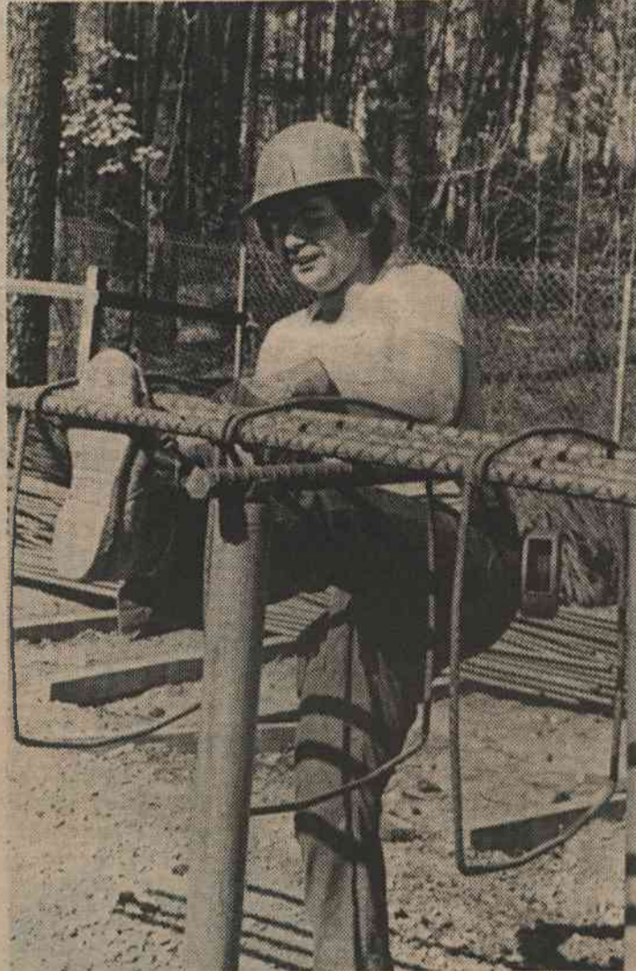
TYING THINGS TOGETHER —Ironworkers Frankie Pittman (left) and James Williams are pictured making reinforcement cages for concrete columns to be used in the construction of the Seeley G. Mudd Building (the medical center's new library) and the Edwin L. Jones Cancer Research Building. Both buildings are scheduled for completion in mid or late 1975. (Photo by David Williamson)
