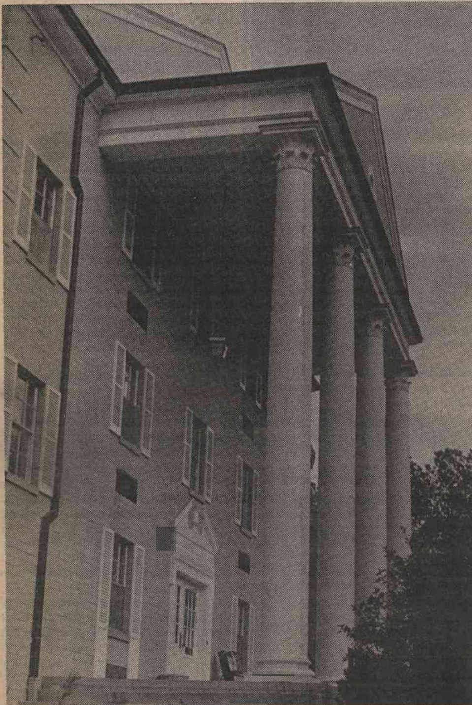
SITE OF NEW 'DUKE WEST' UNIT —This white-columned gray building, located at the corner of Erwin and Moreene roads, is now the home of the hospital's newest inpatient unit — 'Duke West.'
