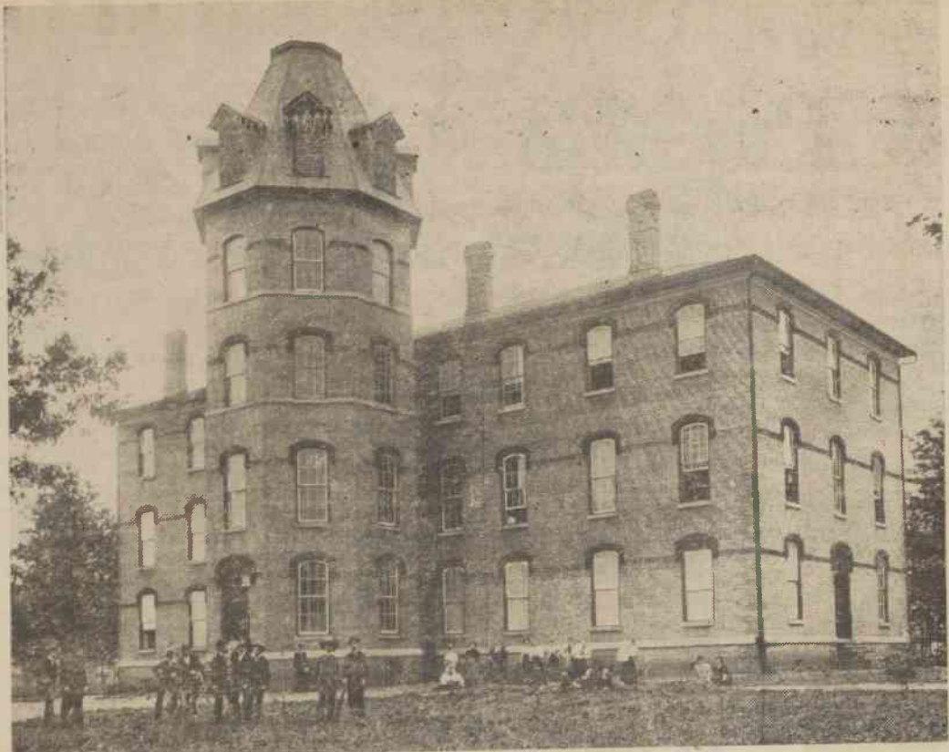
When Elon College opened its doors for its first students on September 2, 1890, the Main Building or Administration Building, oft-times referred to as the "Ad" Building by students of that day, housed the offices, class rooms, library, society halls and even some of the male students. That original Elon College building, which was destroyed by fire in 1923, is pictured above in a photograph taken soon after its completion.
