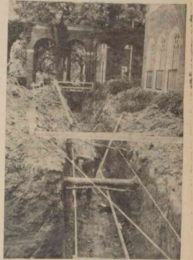
Scenes reminiscent of the World War I trenches in France were seen all over the Elon College campus this summer and have even continued to prevail since the new college year got underway, but both students and faculty endured the inconvenience of hopping ditches and plowing through either dust or mud as they realized that it meant a new heating and hot water system for Elon's campus buildings for this year. The new heat and hot water lines have been installed at a cost of approximately $200,000 and will add much to the comfort of Elon people during the winter months ahead.
