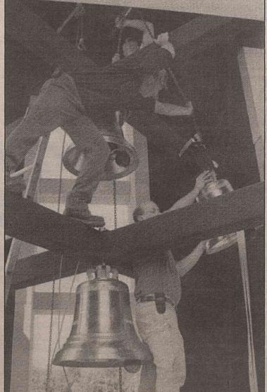
Two weeks ago, the four bells arrived from France. Three workers in the tower used winches to guide the bells into position.
