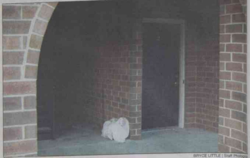
Residents reported a wide array of missing items from liquor to flat screen televisions. This is a second burglary in Trollinger apartments since November.
