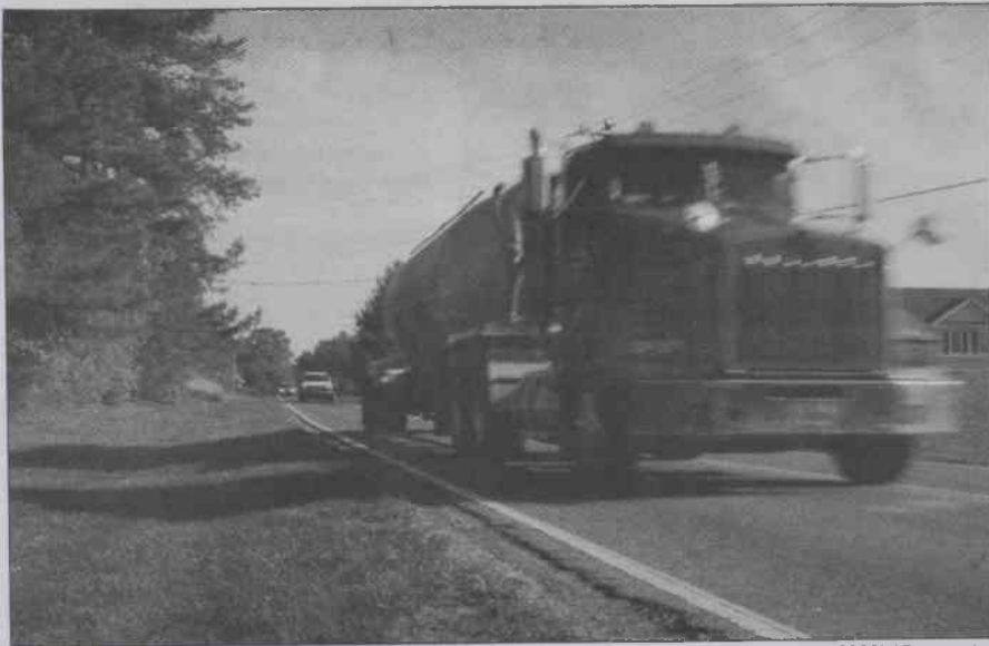
The Cook Road segment of University Drive will be the site of construction starting in the fall that will widen the road and add a bridge over the railroad tracks.
