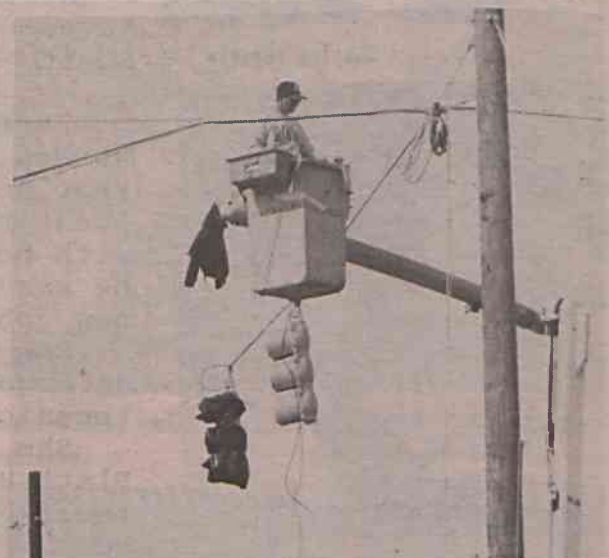
A workman installs a much-needed traffic light.
