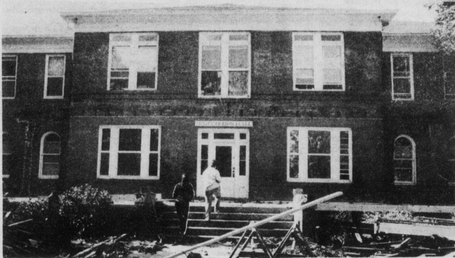
Hobbs porch stripped
