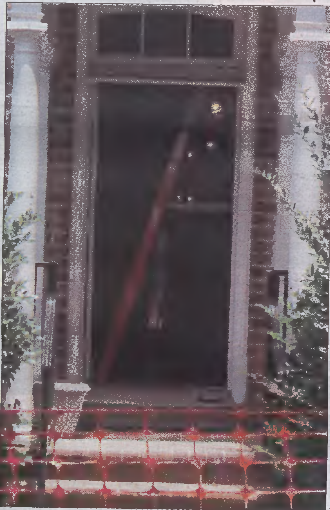
A side door to Archdale Hall is closed for construction. The builders hope to meet LEED gold standards.
