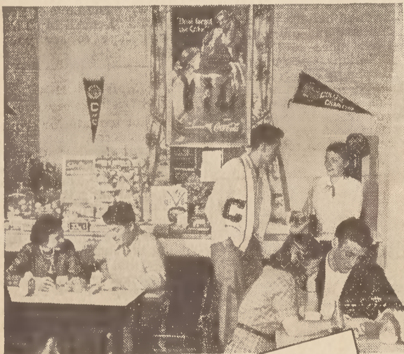
College Canteen College of Charleston Charleston, South Carolina
