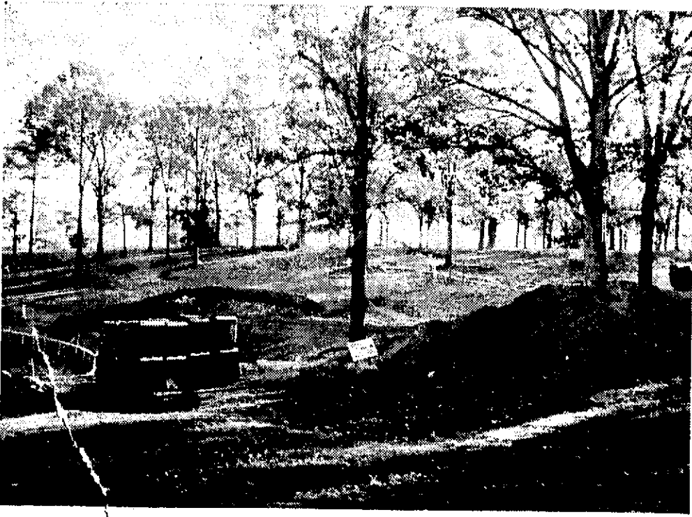
Work on the McIver Amphitheater begins as bulldozers prepare the ground for the pouring of concrete.
